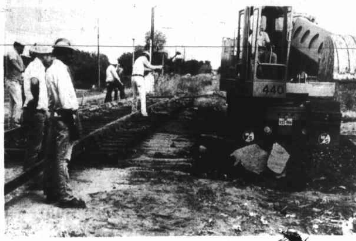
McCarty Street crossing repaired
